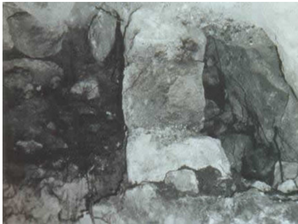
Part of the building's foundation
